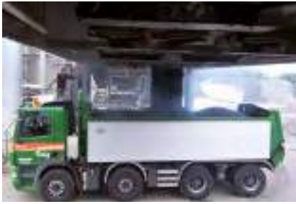
Asphalt and concrete mixing
