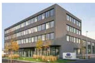
Headquarters of the WAB-GROUP
