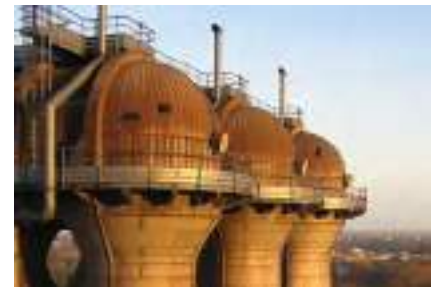
Blast furnace / stove dome
